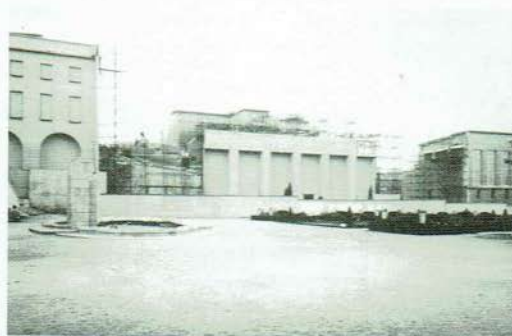
2 Provisionary façade of the Royal Library and the garden of the Mont des Arts. 1963
